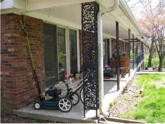
Covered Back Porch along entire back of home!
