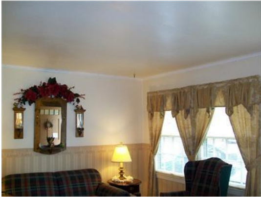
Notice the quality, and the smooth ceiling!
