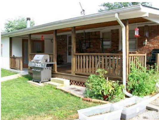
Back View of Covered Deck.
