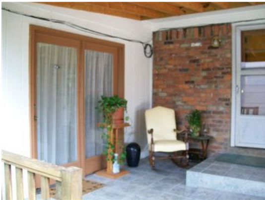
View of Atrium Door from outside.
